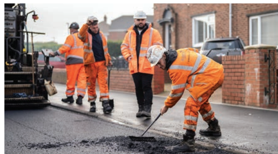
Roads across County Durham being resurfaced with the sustainable asphalt solution.
