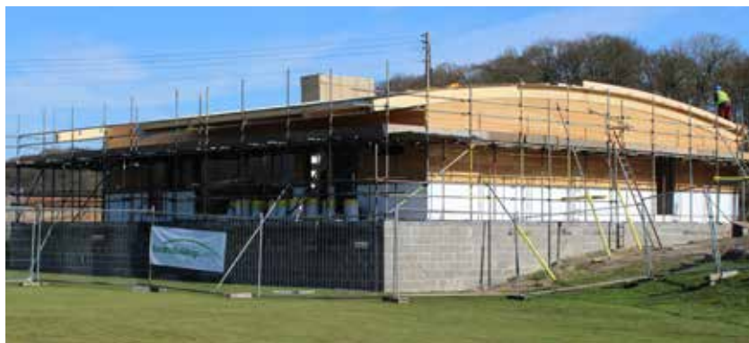
Work continues on the new Mainsforth Cricket Club pavilion with completion expected in mid May.
