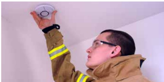
Smoke alarms have saved countless lives over the decades since their introduction.
