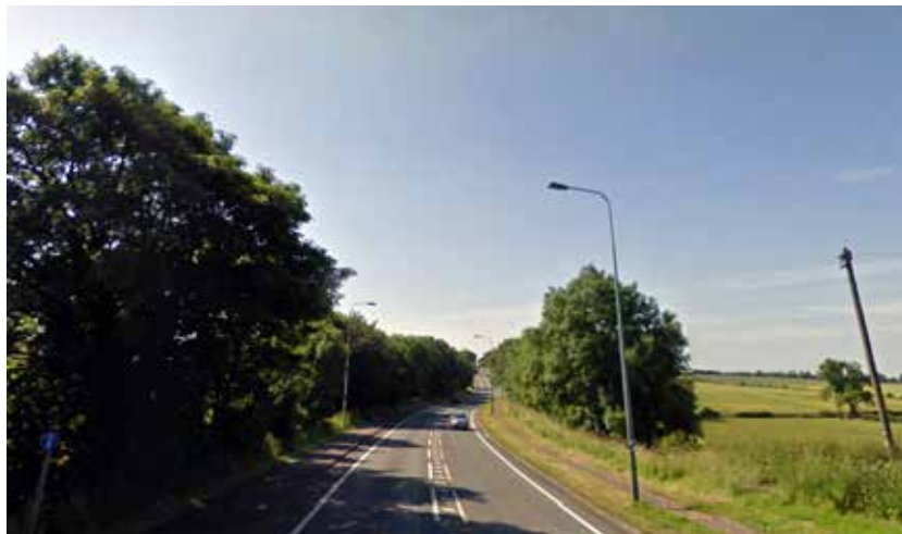
The A167 is a high speed road which has seen a number of accidents and fatalities in previous years in the stretch between Ferryhill and Chilton.
